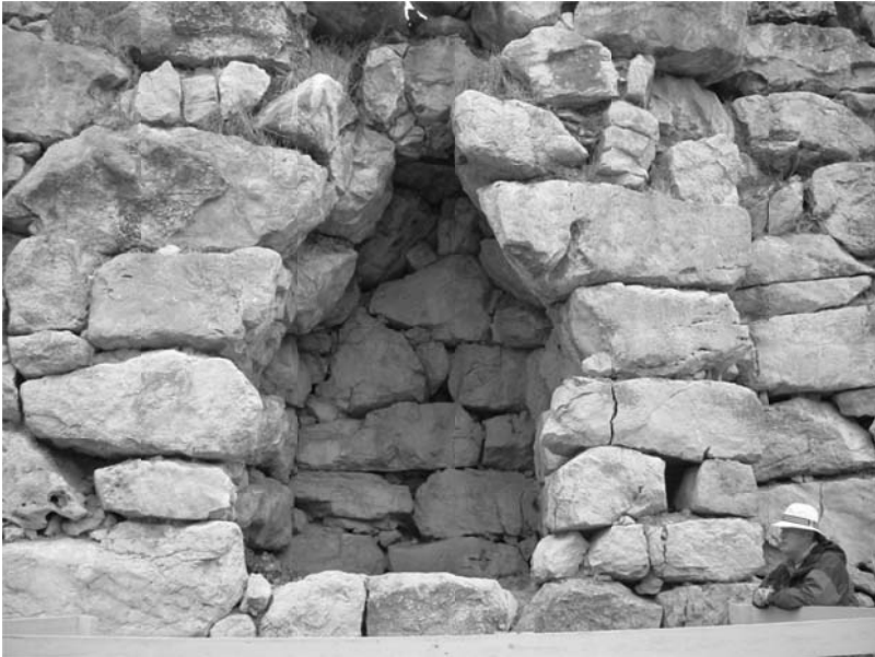
Fig. Intro.1: ‘Cyclopean’ wall at 13 th century BC Tiryns, mainland Greece – main stones filled with smaller ones (person represents scale)
